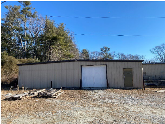
Future home of Hendersonville Connections Center
